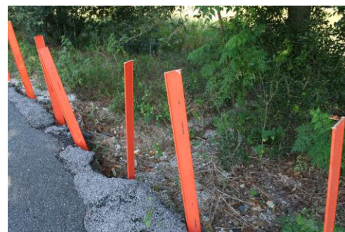
More erosion due to rain washouts.
