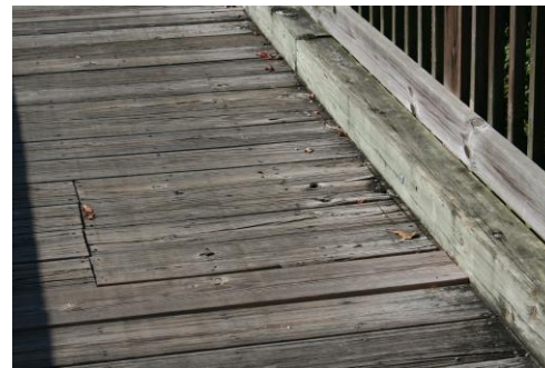
Previous repairs on boardwalk.
