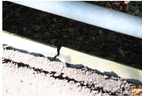
Shift in retention wall due to erosion.
