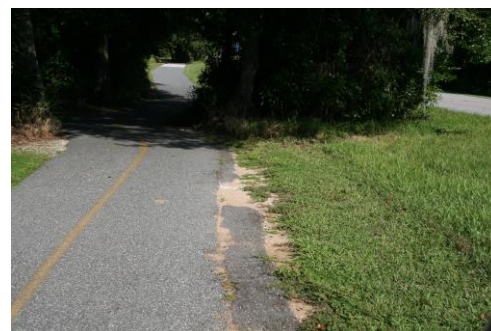
Narrow area of trail and crumbling asphalt.
