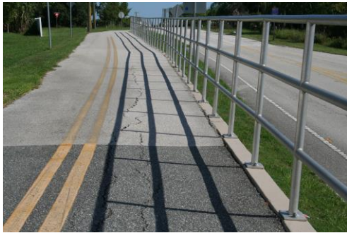
Split asphalt due to weakening of retention wall.
